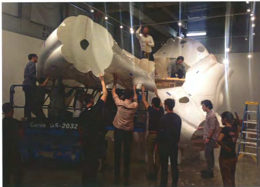
SCI-Arc students lifting one of the nine components into place
