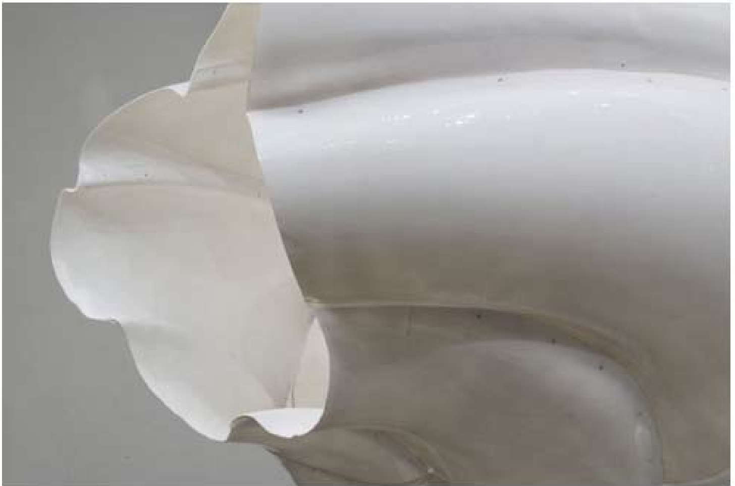
THE 1/8-INCH-THICK STRUCTURE WAS BUILT OF HEAT-FORMED PLASTIC. (JOSHUA WHITE)
